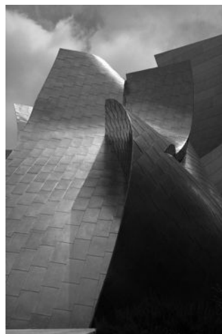
The Founders Room at the Walt Disney Concert Hall, Los Angeles, designed by Frank Gehry.
